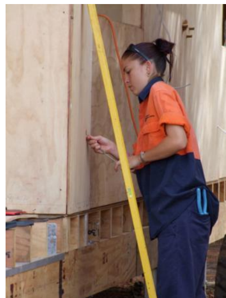
Electrical wiring in progress
