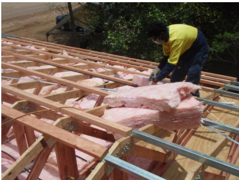
Roof insulation being installed
