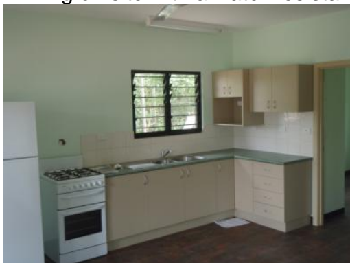
Finished interior – Kitchen
